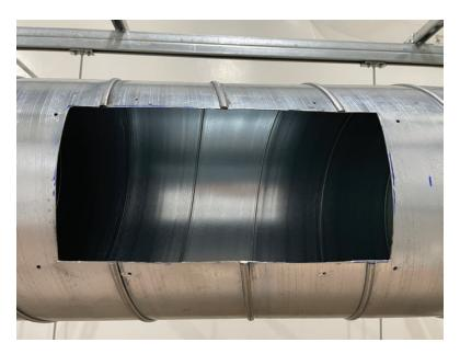
Step 3: Insert the spiral duct grille in the duct opening.
